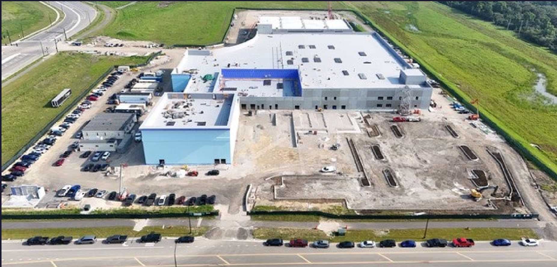
Hollywood Casino Joliet (new site in development)
